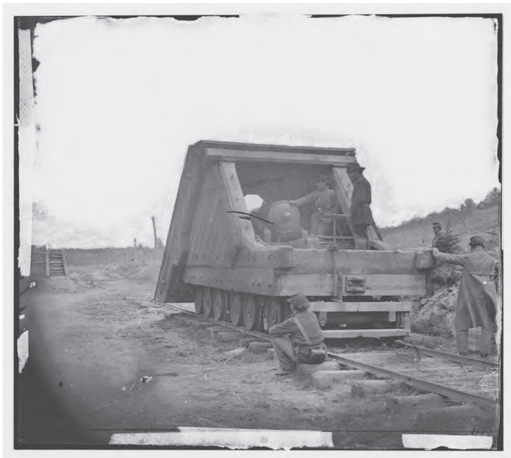
New and more destructive warfare technology emerged during this time that used discoveries and innovations in other areas of life, like transportation. This photograph shows Robert E. Lee's railroad gun and crew used in the main eastern theater of war at the siege of Petersburg, June 1864–April 1865. Petersburg, Va. Railroad gun and crew , between 1864 and 1865. Library of Congress.
